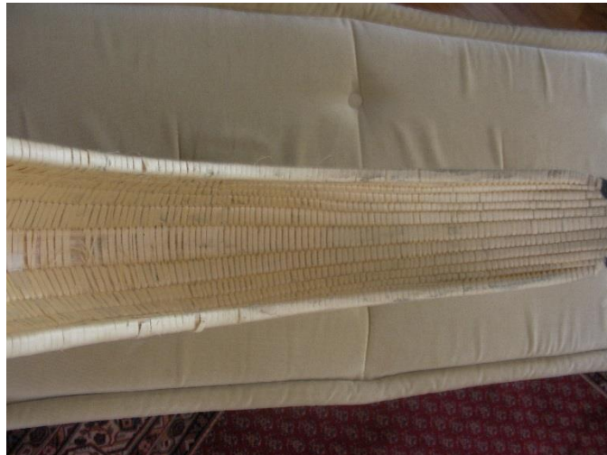
The frame tape has been removed and reed damage has been exposed.
